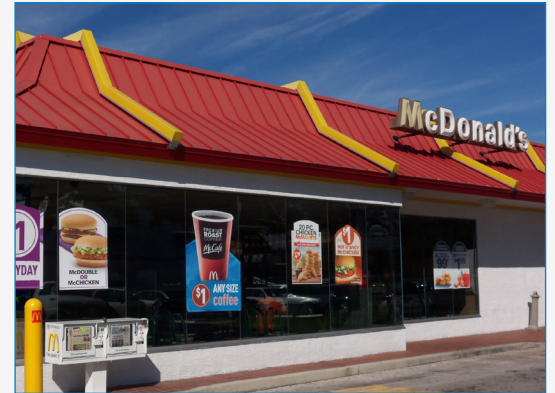
The independently owned McDonald's in Piscataway installed LEDs, replaced T12 fixtures with T8 lighting and installed five new HVAC units. The energy efficiency improvements are expected to save $9,481 each year. Photo by Daniel Oines.
